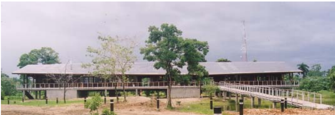
The new lab facility at Bocas del Toro, Panama. To the left of the bridge are two large labs for groups of researchers as well as several smaller labs for individual long term researchers. To the right of the bridge is an office and a library. (Photo by Geoff Keel)
